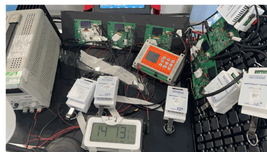
Figure 5 Original supply/interface and monitoring connections, source p. 92.
